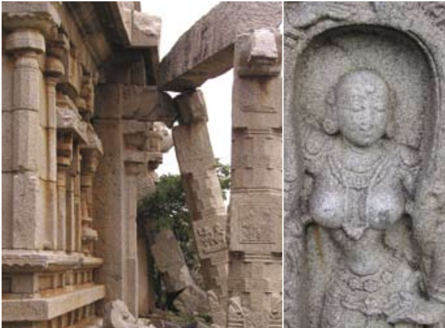
Left: Collapsing entry gateway.
