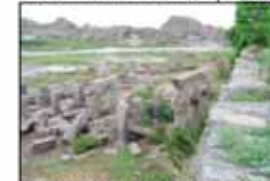
remnants of bridge abutting the embankment wall
