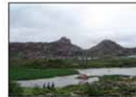
remains of old stone bridge across the tungabhadra
