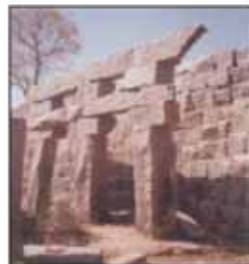
monolithic granite pylons of the bridge abutting the embankment of the chandramauleshwar temple
