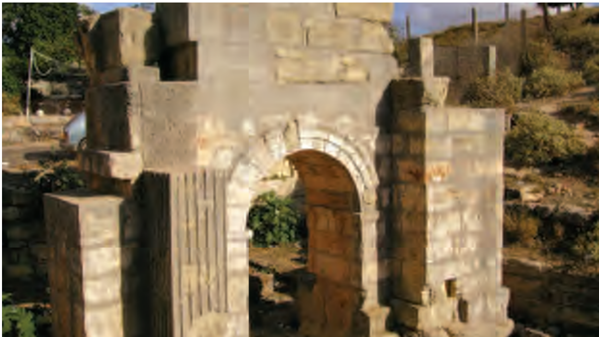
In Cyrene, Libya, a UNESCO World Heritage Site, Portland cement and rebar is used to patch together ancient monuments even today. Inappropriate reconstructions and unauthentic restorations for tourism are one of the most severe causes of loss and destruction to global heritage sites. Photo: GHF
