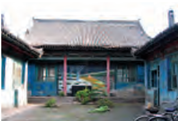
Top: Mijia Xiang Courtyard after GHF restoration; Middle: During restoration; Bottom: Before restoration. Photos: GHF
