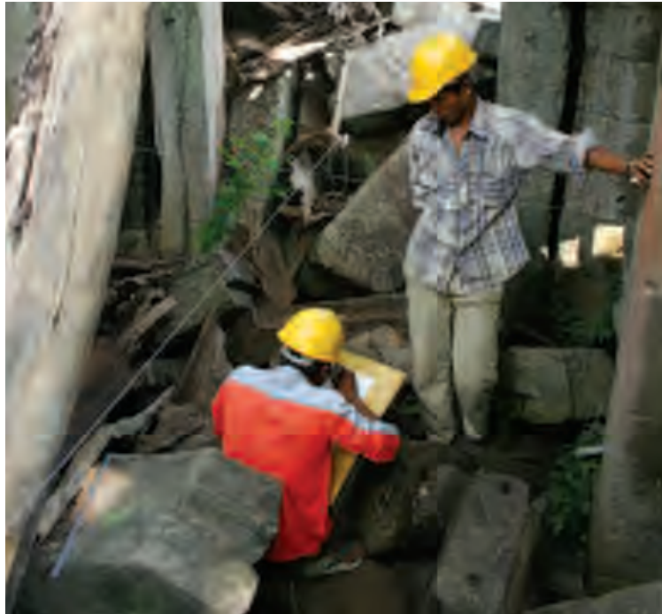
Facing page, top: In Banteay Chhmar, GHF is working with an all-Khmer conservation team to stabilize and scientifically restore the Citadel of the Cats. Photos: GHF
