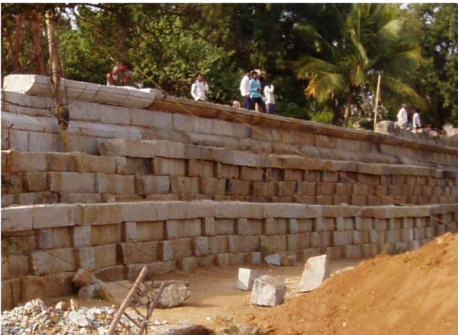
Restoration of embankment wall. Photo by James Hooper
