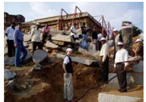
Conservation of the Chandramauleshwar Temple underway. Photo by James Hooper
