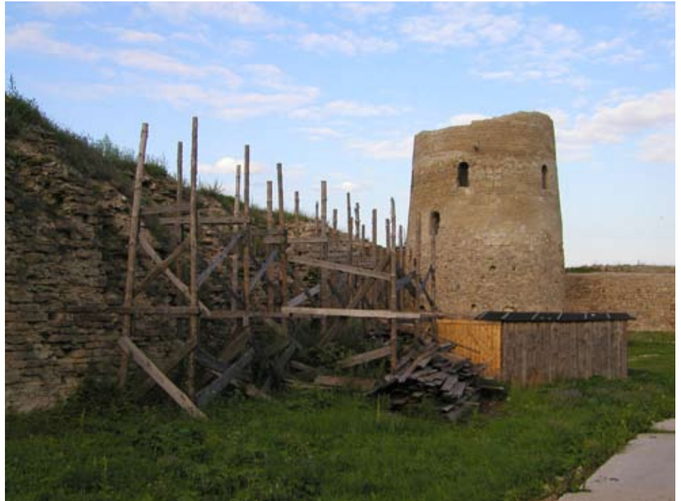
Restoration of interior wall. Photo by John Hurd
