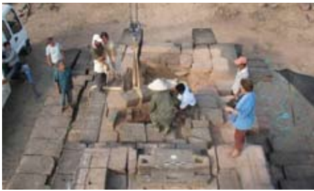
Restoration and stabilization efforts on Nandin Hall. Photo by © Leric Institute
