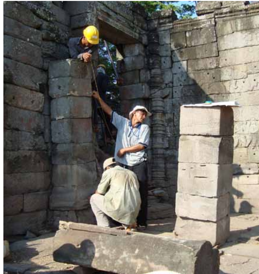
Below: Work continues on the Southeast sector of Bas Relief East Enclosure Wall Banteay Chhmar, Cambodia. © GHF
