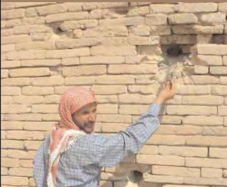
Damaged from shrapnel Iraq World Heritage Site
