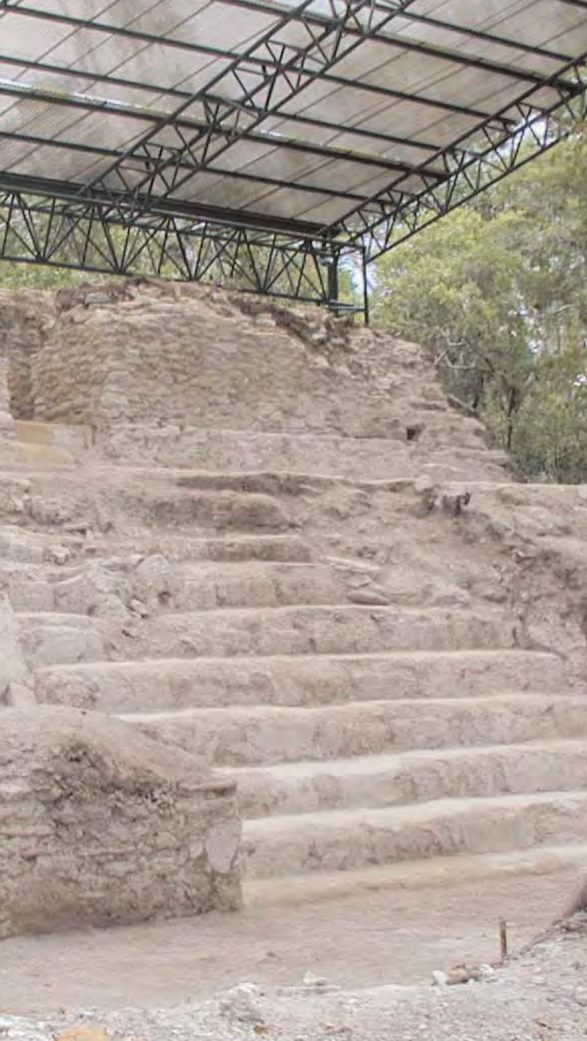
GHF sponsored conservation technology includes roofing to protect Preclassic Maya monuments. Mirador Basin, Guatemala
