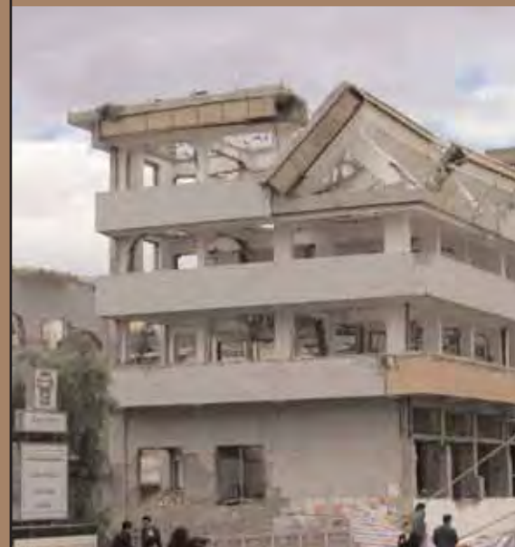
Removal of modern building Lijiang Ancient Town, China
