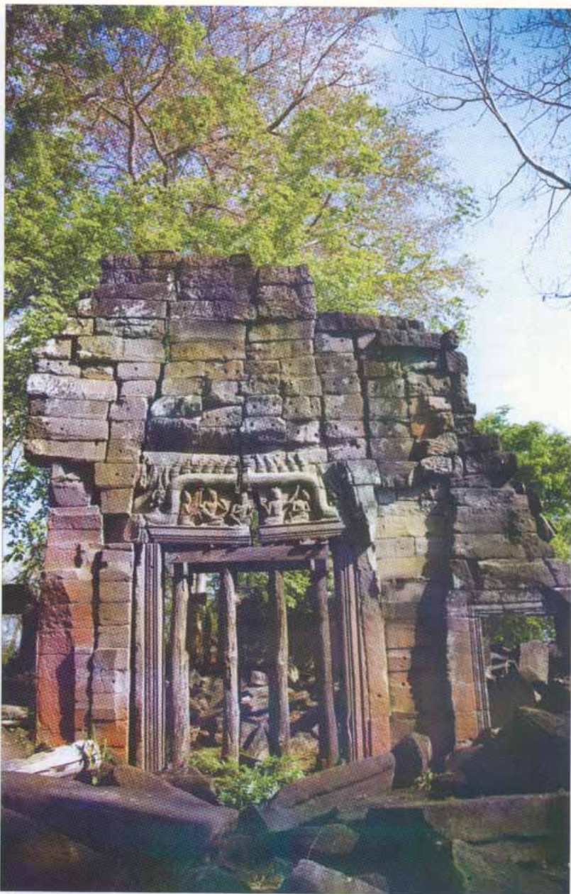
Emergency measures were used to prevent the collapse of the door to the Hall of Dancers at the Banteay Chhmar monument.
