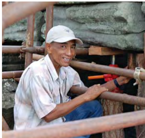
Erecting support scaffolding at Banteay Chhmar, Cambodia. Photographer: Dan Thompson
